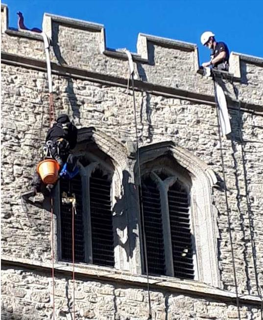
For some time now, crows have been forcing their way past the installed chicken wire and into the tower to nest and roost. Not only was this distressing to the birds since they could become trapped, but it also created fouling in the tower and damage to the bells.
